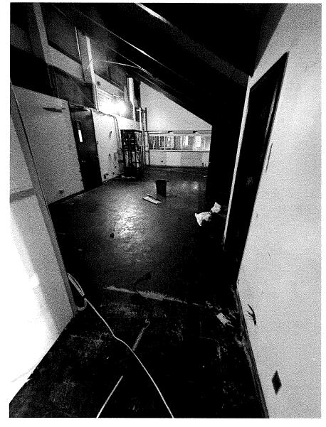
Abatement of floor tile in the 2<sup>nd</sup> Floor office and staircase completed successfully by Unitech. JC Broderick provided monitoring and Stalco installed new hallway on the second floor and temporary completed their 24-hr. air quality testing. partition walls to accommodate phase 2.
