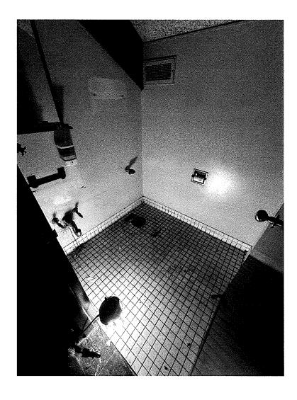
Hirsch removed all existing fixtures and rough plumbing below the floor slab and capped existing drain lines. CDJ removed the existing circuit power to the bathrooms and provided temporary lighting for contractors.
